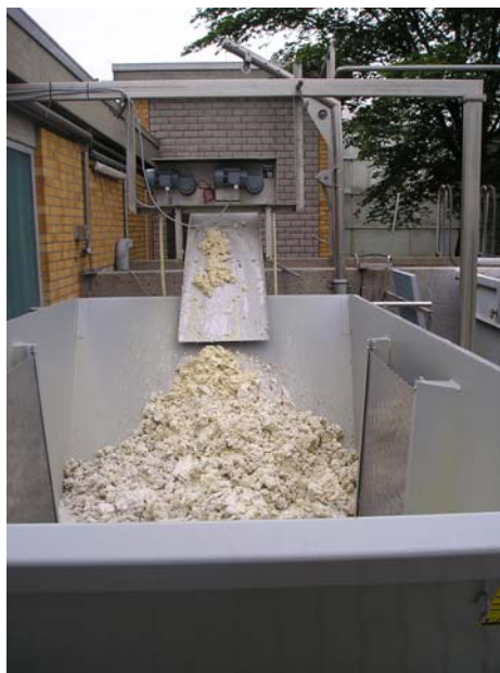
Container with dewatering sieves at each sides of the container
